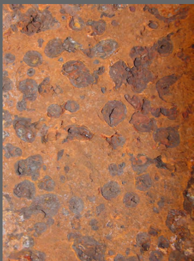
Localised corrosion for high levels of salt
